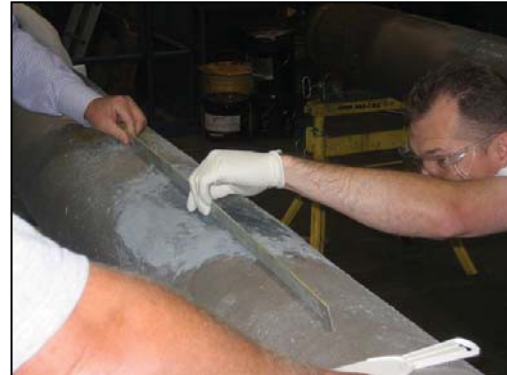
Fig. 4 – Use a straight edge to confirm evenness.
