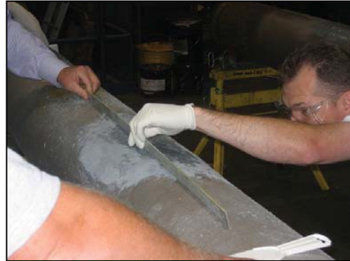
Fig. 4 – Use a straight edge to confirm evenness.
