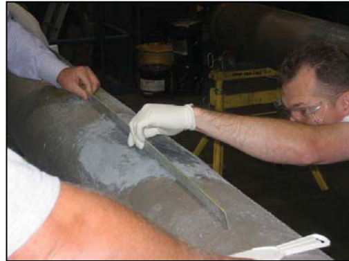
Fig. 4 – Use a straight edge to confirm evenness.
