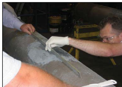
Use a straight edge to confirm evenness
