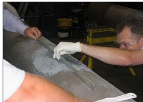
Use a straight edge to confirm evenness
