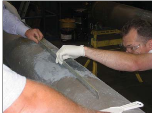
Fig. 4 – Use a straight edge to confirm evenness.
