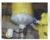
Conforms to ASME PCC-2 Article 4.1 Nonmetallic Composite Repair Systems for Piping and Pipework: High Risk Applications
