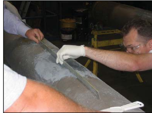
Fig. 4 – Use a straight edge to confirm evenness.
