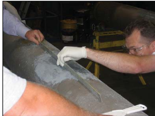
Fig. 4 – Use a straight edge to confirm evenness.
